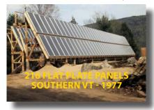
For best results, the panels should be mounted on a south-facing location, within 30° of true south.
